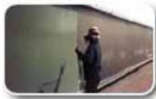
High Performance Coating & Lining
